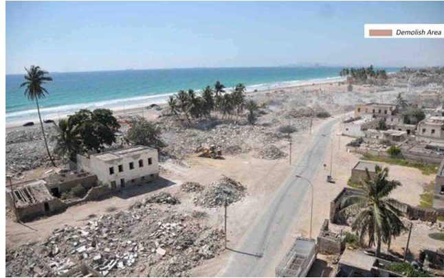
Figure 3 : Figure xx: the project phase one: The Demolishing Area, Source: (Twitter @omanprojects, 2015)
