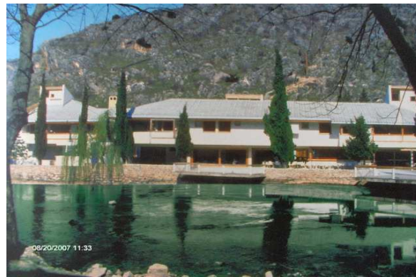
Figure 2. Hotel Bregava hovering above the water (from old hotel brochure)
