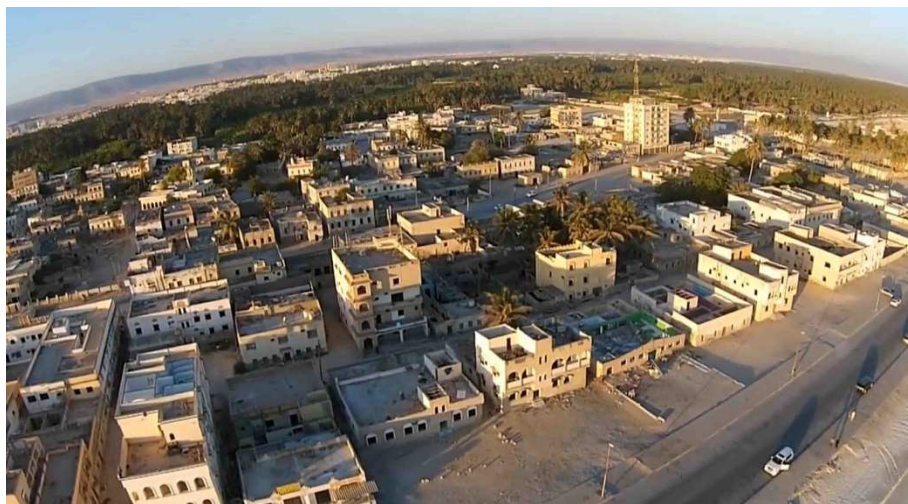
Figure 1 1: The old district of Al-Hafa (demolish area), Source: (Alwadi, 2014)
