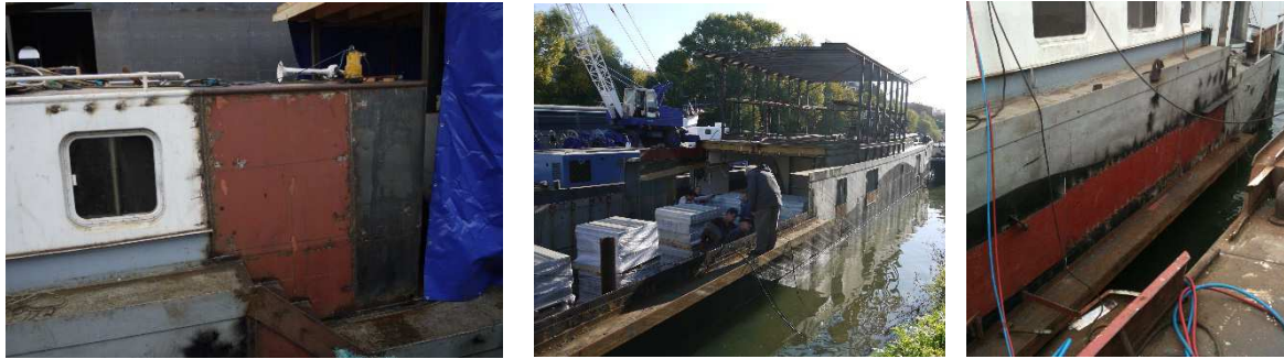
Figure 7. Feldzer T.( 2014), India Tango Boat, Site construction, Paris. Expansion, raising, enlargement, shortening and cutting of a Freycinet péniche
