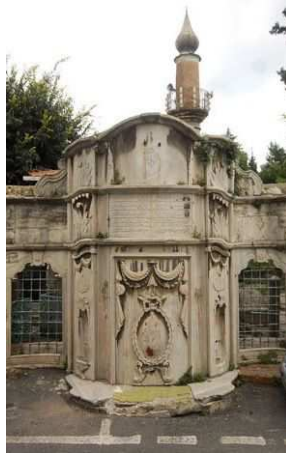
Figure 6. Water faucet on the outer wall of the Fevziye mosque in Istanbul, Turkey ( https://tr.pinterest.com )
