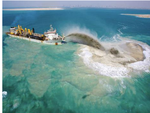
Figure 8. Process of ‘rainbowing’ to deposit the sand above sea level.
