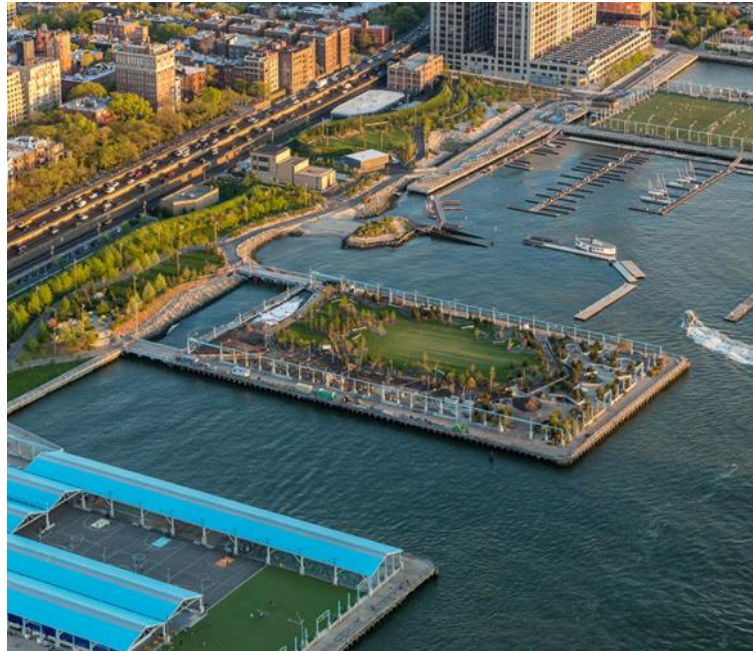
Figure 12. Brooklyn Bridge Park, Pier 3 (Franklin, 2018).
